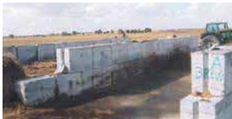
Concrete block bunkers
